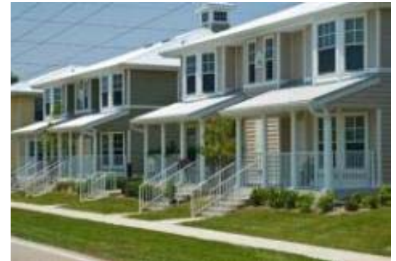
GULF BREEZE APARTMENTS: NEW RESIDENTIAL DEVELOPMENT SET ON A TRADITIONAL STREET GRID
